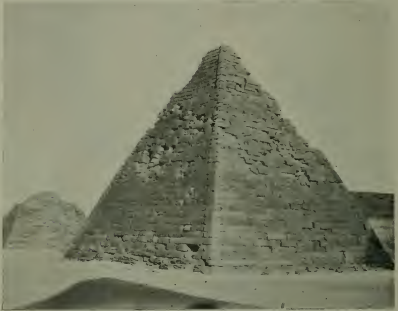
A PYRAMID AT GEBEL BARKAL, SHOWING THE ARRANGEMENT OF THE STONES AT ONE CORNER.
